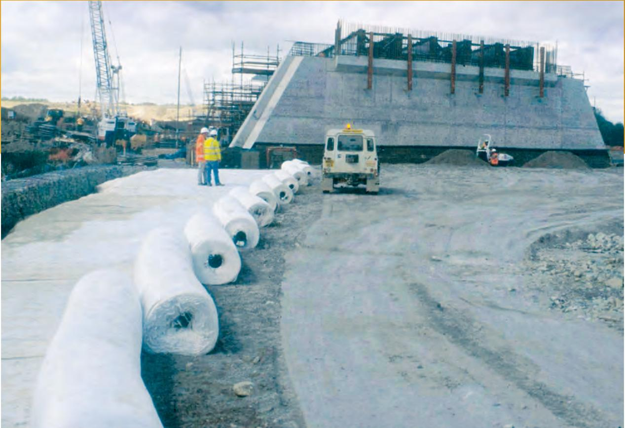
*Tensar Basetex in a Tensioned Membrane Load Transfer Platform supporting an embankment for high speed railway.*
