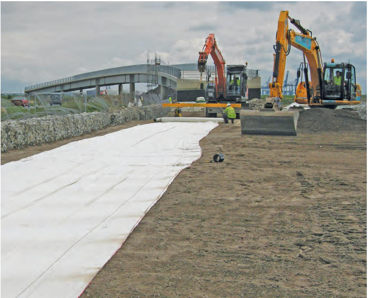
*Installation of Basetex in a Tensioned Membrane Load Transfer Platform over bored piles on the A228 highway embankment over alluvium in Kent.*
