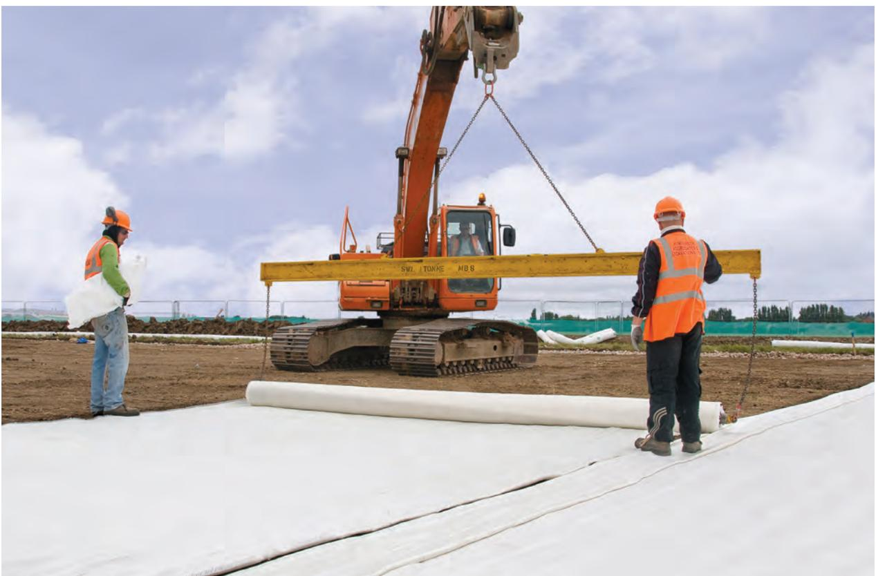
*The standard roll size of Basetex is 4.4m wide x 100m long which allows very rapid installation.*
