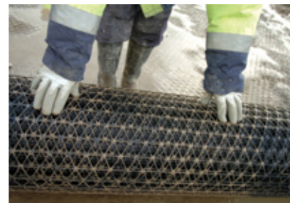
Standard roll sizes make TriAx Geogrid easy to maneuver with minimal waste.
